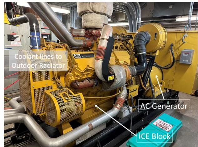
Figure 1: Example test bed enclosed, unheated, 1MW EPS.
