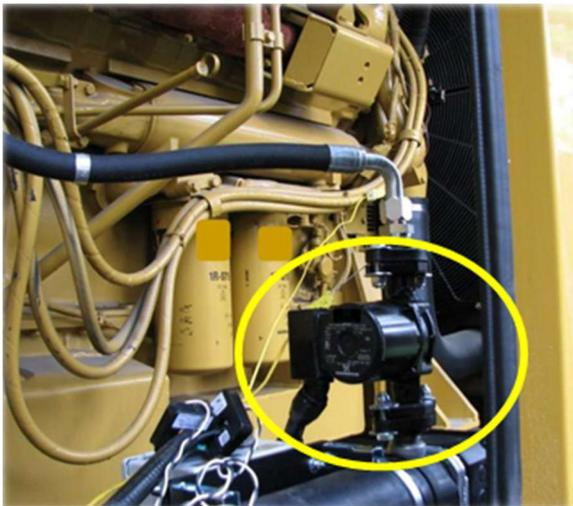
Figure 2: Examples of an ICE heater in an outdoor application.
